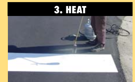
Heat HotTape™ with a propane heat torch such as the Magnum Heat Torch then chisel test to ensure proper bond.
