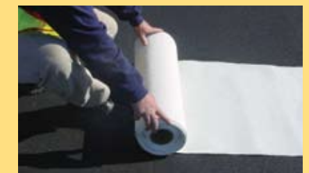
Unroll or lay out the flat sheets of material as desired for particular marking.
