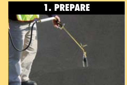
Clean the surface to remove any debris. Preheat the pavement surface to a minimum of 300° F.
