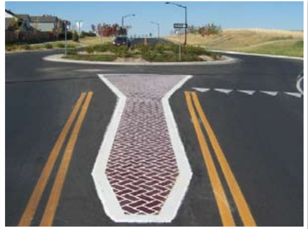
Traffic islands at these roundabouts in Erie, CO are made from the DecoMark® Herringbone surface pattern. Emergency response teams appreciate the use of preformed thermoplastic as an alternative solution because of the low profile.
