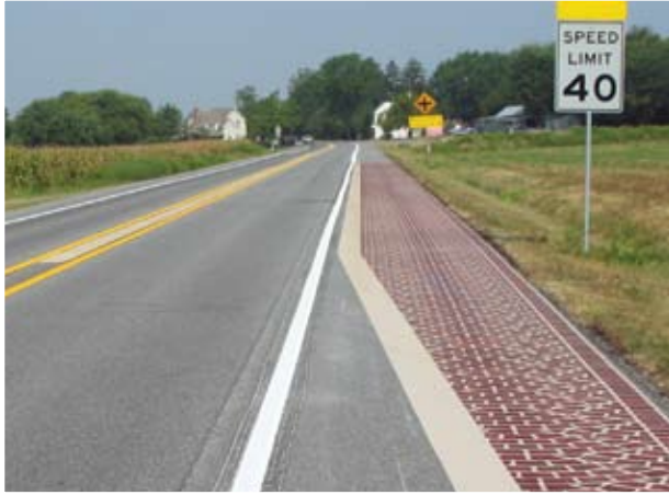
The DecoMark® Cobblestone surface pattern used with a 12" sand-colored border to simulate a drain pan effect. This traffic calming effect was used as a supplement to the newly-posted speed limit to slow drivers on a rural road in Starr, MD.
