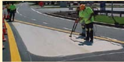
Sand-colored PreMark® is supplied in 2'x3' sheets, cut on-site and heated to the surface with a propane heat torch to create the look of splitter islands.
