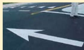
Regulatory markings such as arrows, yield markings (Shark's Teeth), and lines were applied using PreMark preformed thermoplastic to complete this project...all in a day's work!
