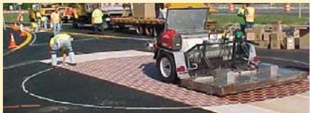
The center of the roundabout is the DecoMark® Courtyard surface pattern using brick-red and sand colored preformed thermoplastic (detail shown at right). Shown above, a large radiant heater is used for larger application areas.
