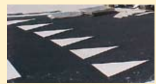
Regulatory markings such as arrows, yield markings (Shark's Teeth), and lines were applied using PreMark preformed thermoplastic to complete this project...all in a day's work!
