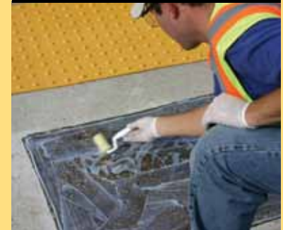
Remove debris from surface. Ensure no moisture is present. Apply TopMark Sealer and Bonder Paste.
