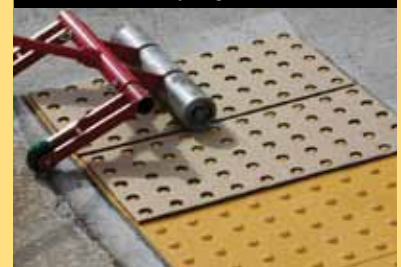
Place holed corrugated inserts on heated portion of domed sheets and roll. Remove excess bonder paste from edges before heating just the edges of the entire application.
